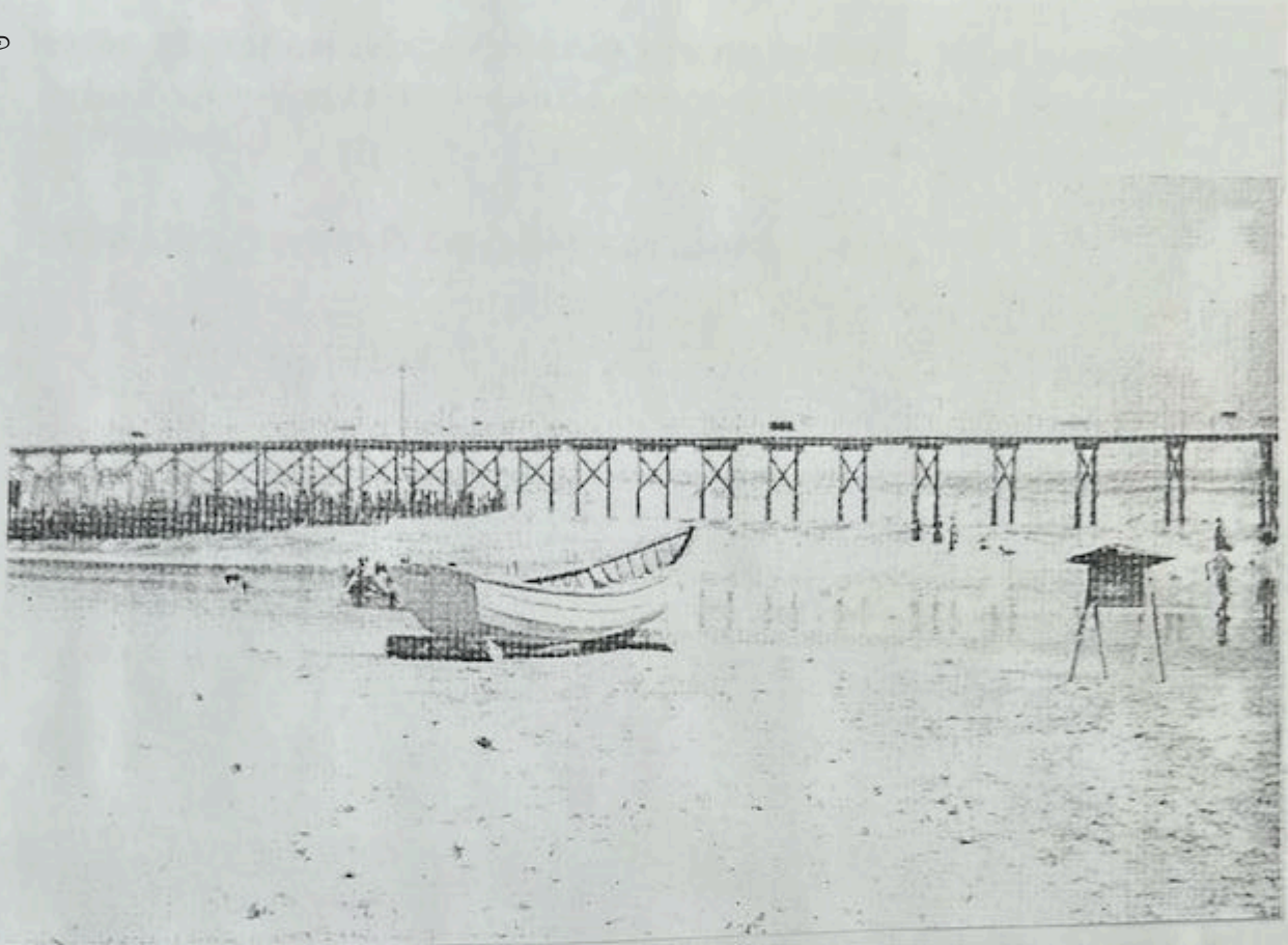
1919- The first fishing pier was built and completed on July 14th at the cost of $6400.
